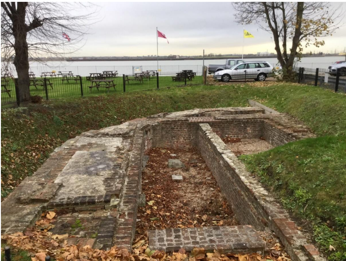
Plate 5.6 Gravesend Blockhouse (SM16) looking north towards the River Thames
