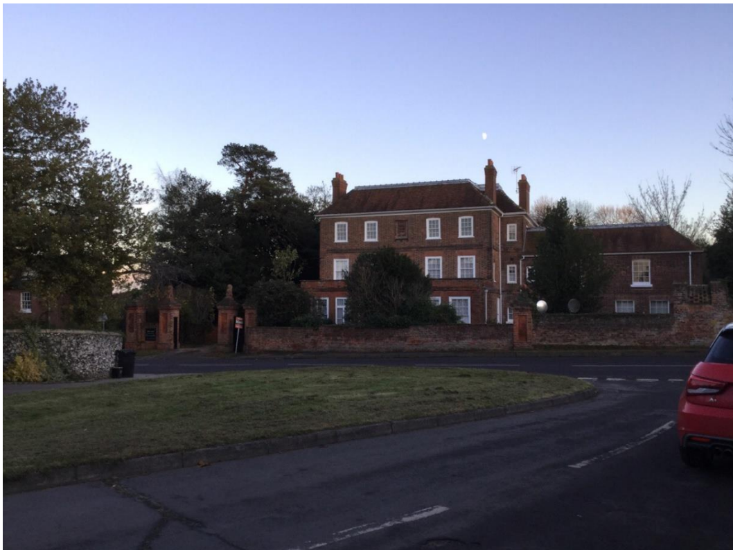
Plate 5.5 South-east view towards higher status building of Pipes Place (LB15) and Front Garden Wall and the Gate Piers to Pipes Place (LB16)
